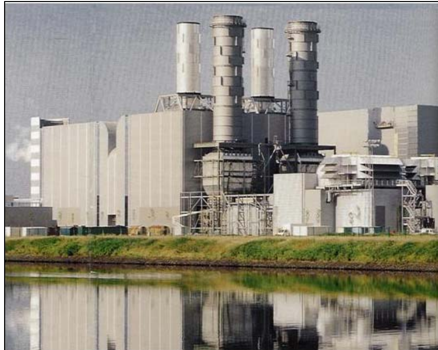
Figure 7.8: Recently built gas turbine combined cycle power plant in Belgium
